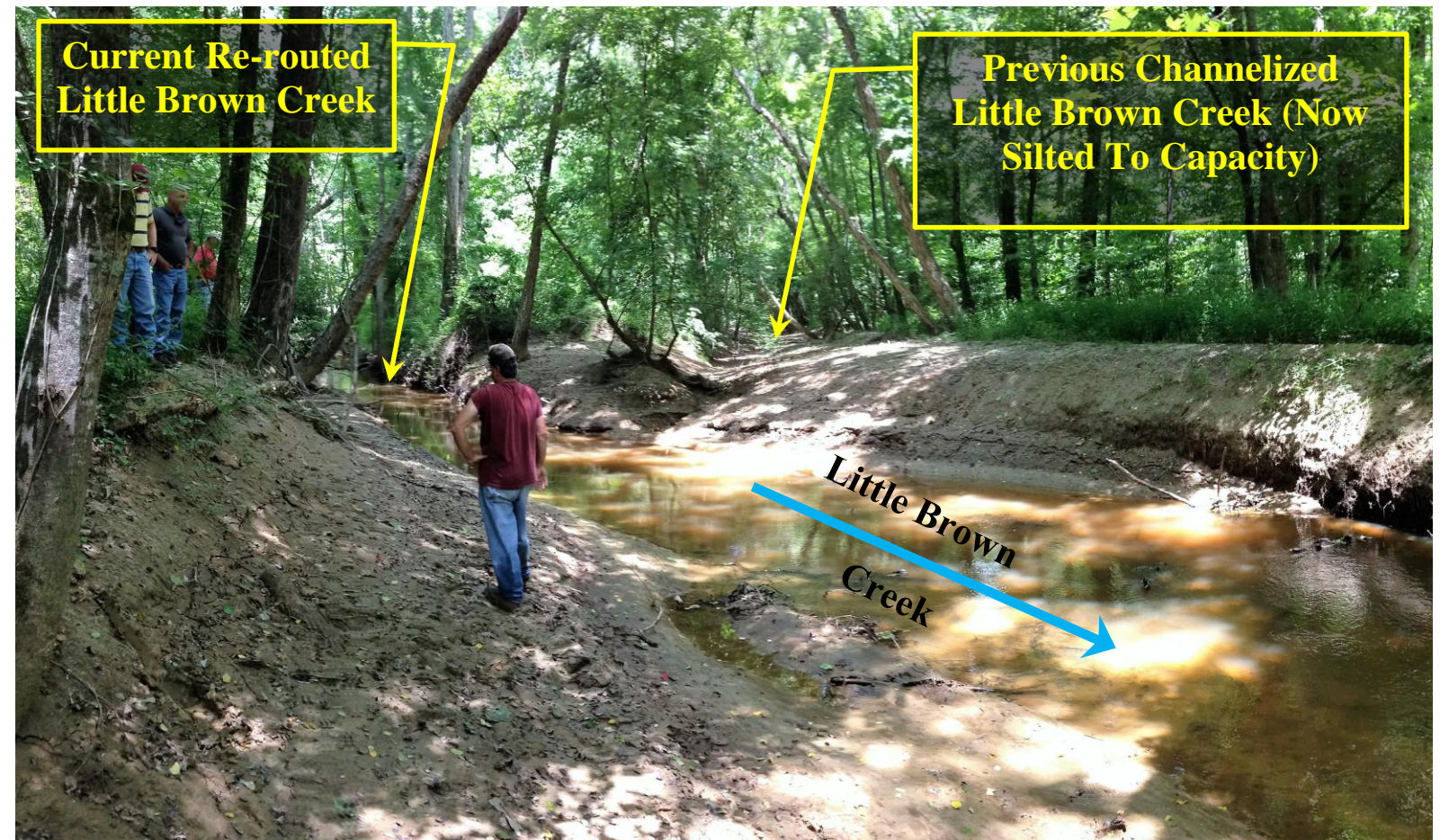
Photo 2: Area of Major Breach, View to South/Southwest (Approx. 200' N of Confluence)
