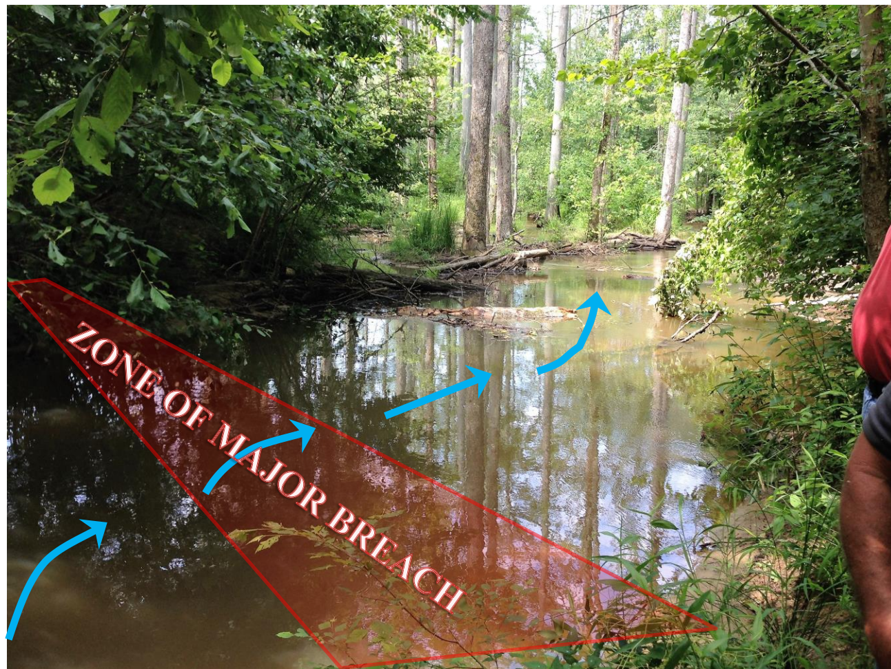
Photo 1: Area of Major Breach, View to South/Southwest, 34°27'09N / 88°25'21"W
